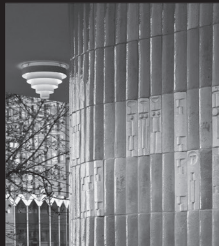
PAWILON CEPELIA CEPELIA PAVILION
